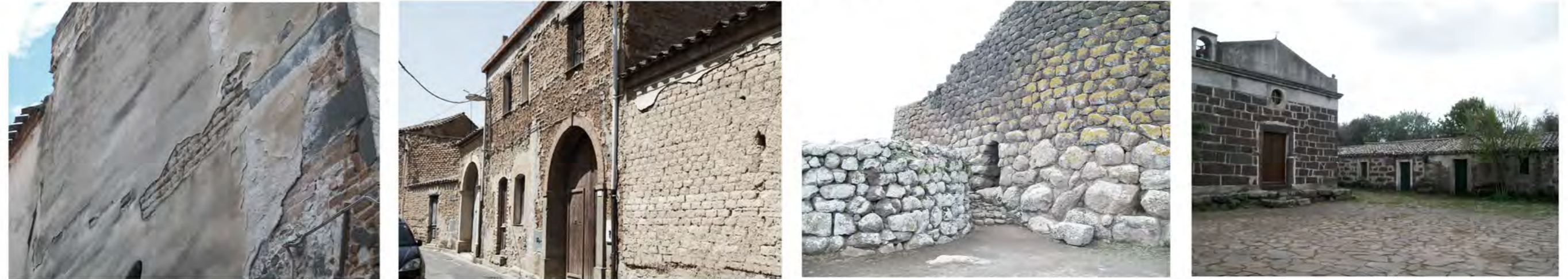
Buildings in Oristano, made by sundried earth blocks
