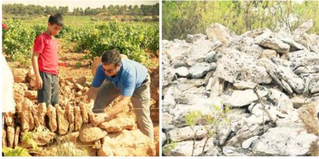
Although stone wall may seem a simple construction, it performs several interesting features. It functions as retaining walls for agricultural terraces **e 11-12-13'**. It drains stormwater and prevents erosion. **d 5-6-7'** It is built with stones taken from the fields. **a 15'** It allows animal shelters and growing plants inside its joints. Thus, it becomes a reliable biological corridor between the fields. **b 1'** In short, it is an essential element of the cultural landscape. **c**
